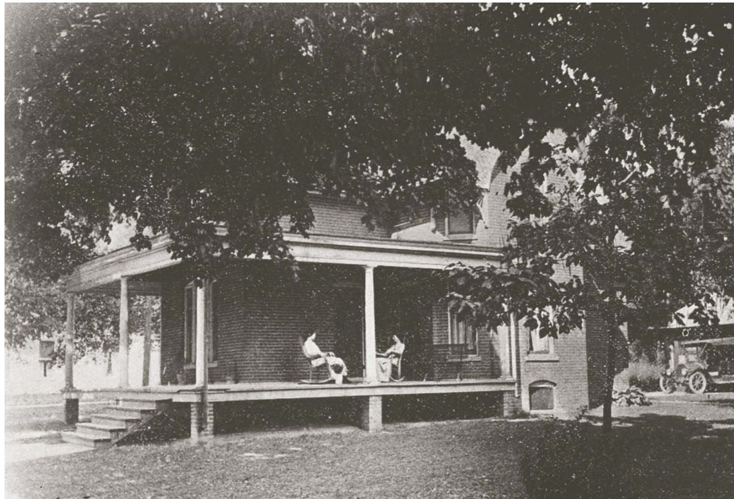
1. Lembke’s Home at 304 N Morgan Boulevard • Built circa 1892, image courtesy of Steven Shook
