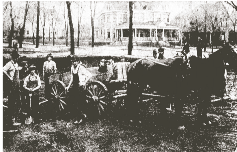
Hotel Lembke Construction begins on the southwest corner of the intersection of Jefferson and Lafayette Streets, circa 1919
